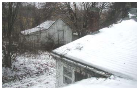
Milk House, View to the North
