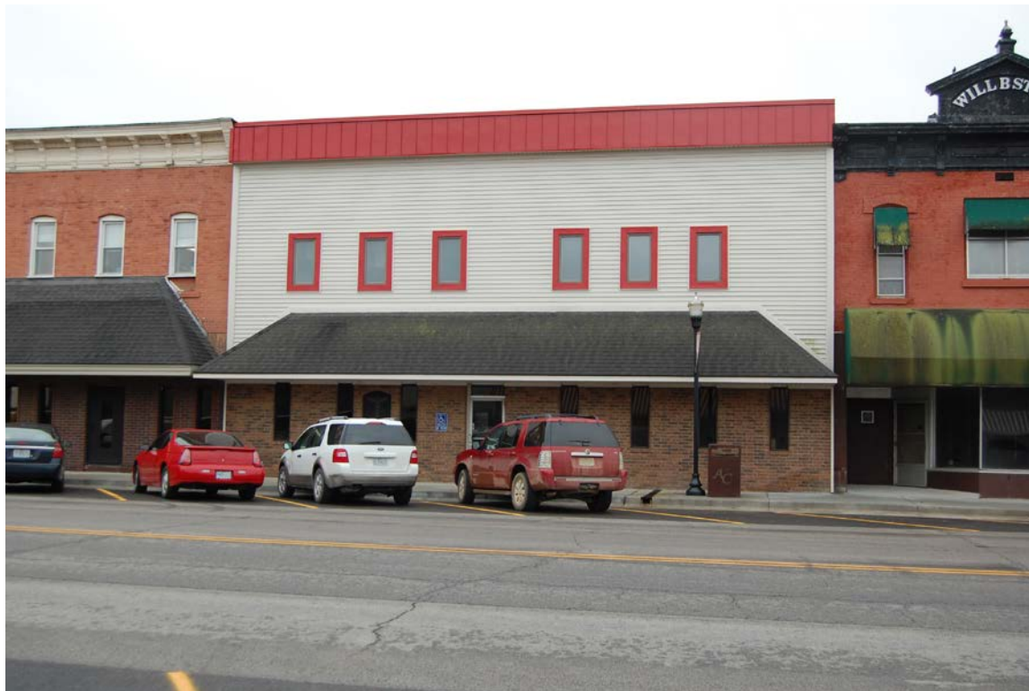
Figure 9. 118-120 W. 4th Street has been altered on lower and upper floors. The building is a non-contributing resource in Appleton City's downtown commercial district. View is south (Photo: Ruth Keenoy, 16 February 2018).
