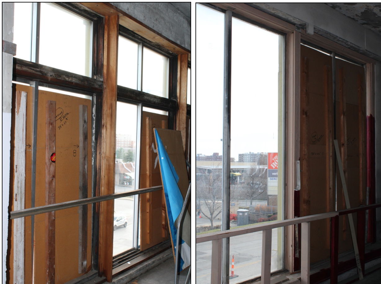
Figure 27: (Left) Interior, second floor; detail of original curtain wall system, with inset second curtain wall components and mural board panels, 2022 (Right) Interior, third floor; detail of original curtain wall system, with inset second curtain wall components and mural board panels, 2022.
