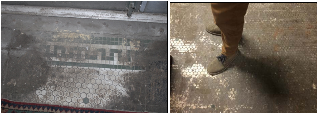
Figure 29: Original decorative tile outlines the showroom area at the northeast portion of the first floor, 2022.
