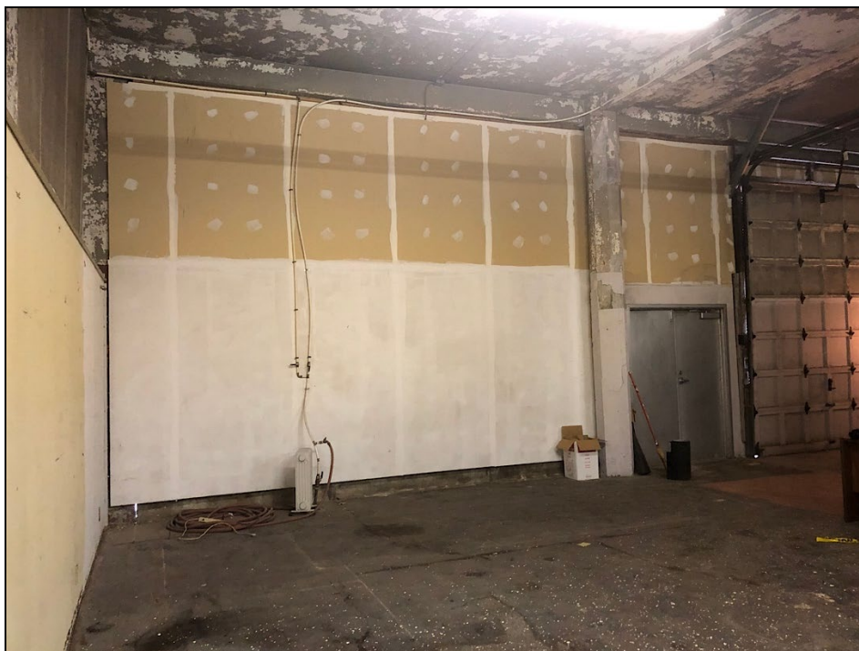
Figure 26: Interior, first floor; view facing east. Source: Kelsey Lutz, photographer.
