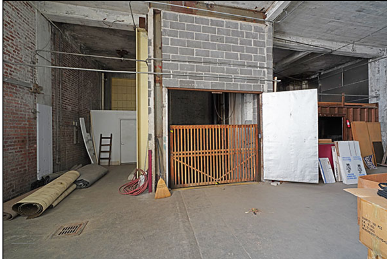
Figure 28: The original freight elevator, located centrally along the western wall of the building, 2022.
