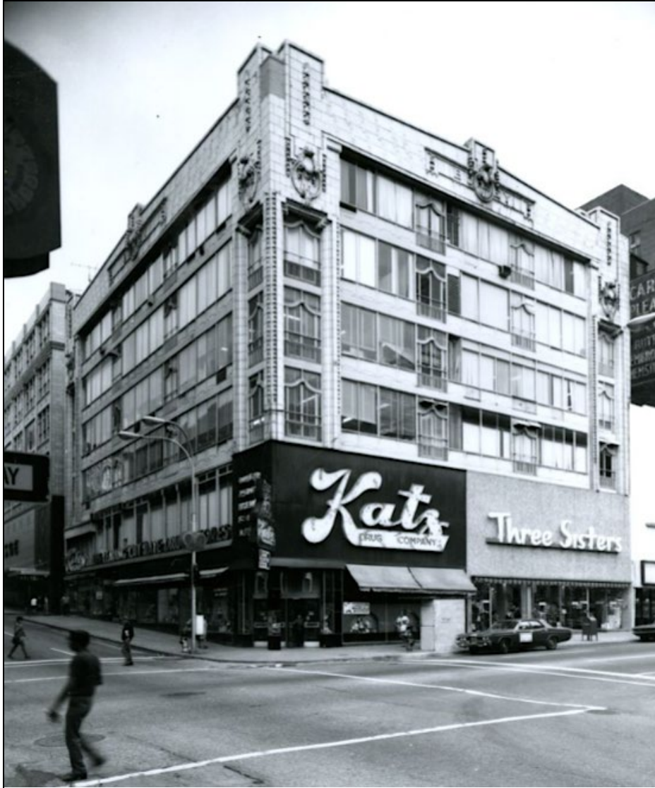
Figure 24: The Boley Building, 1130 Walnut Street, Kansas City, Missouri, photo c. 1970s.
