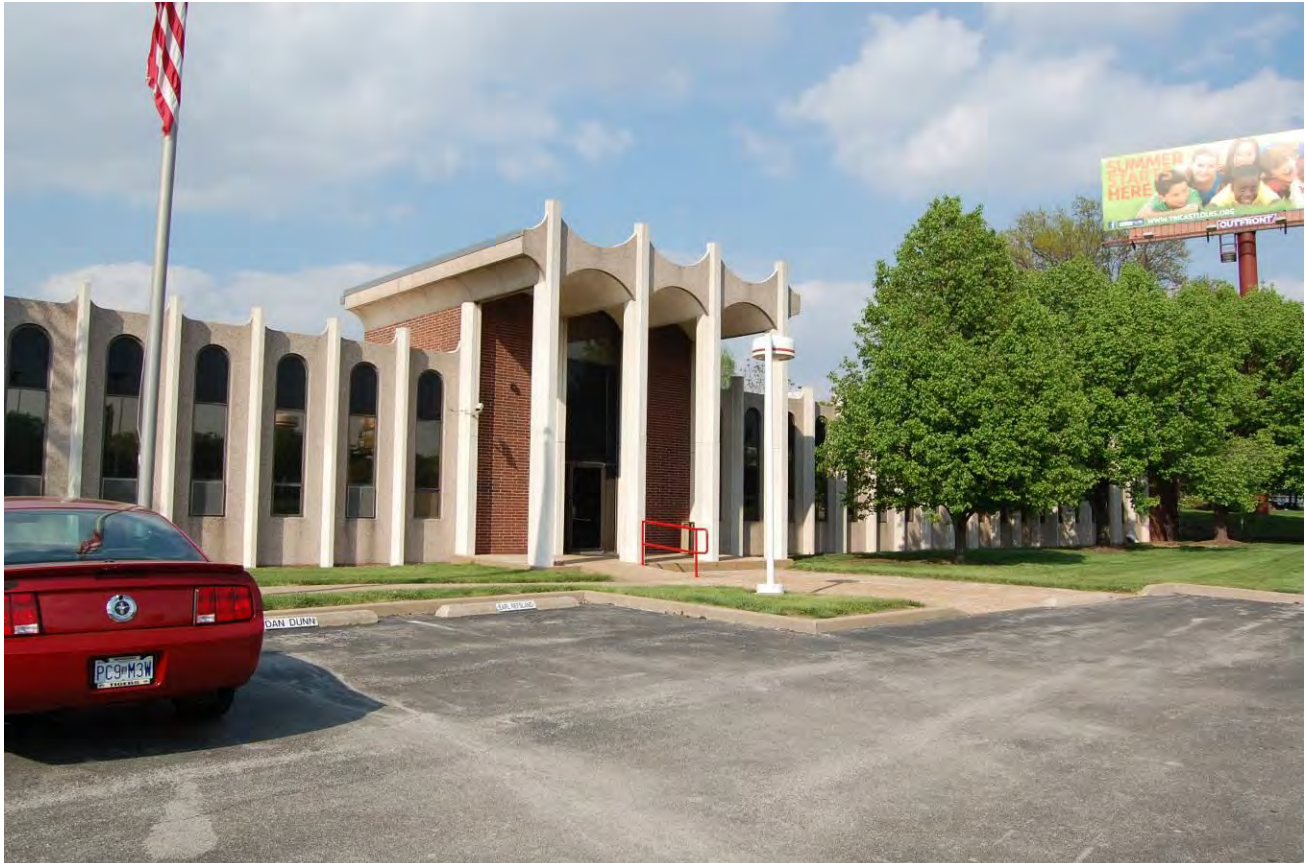
Figure 13. 1720 Sublette Avenue, view is northeast.
