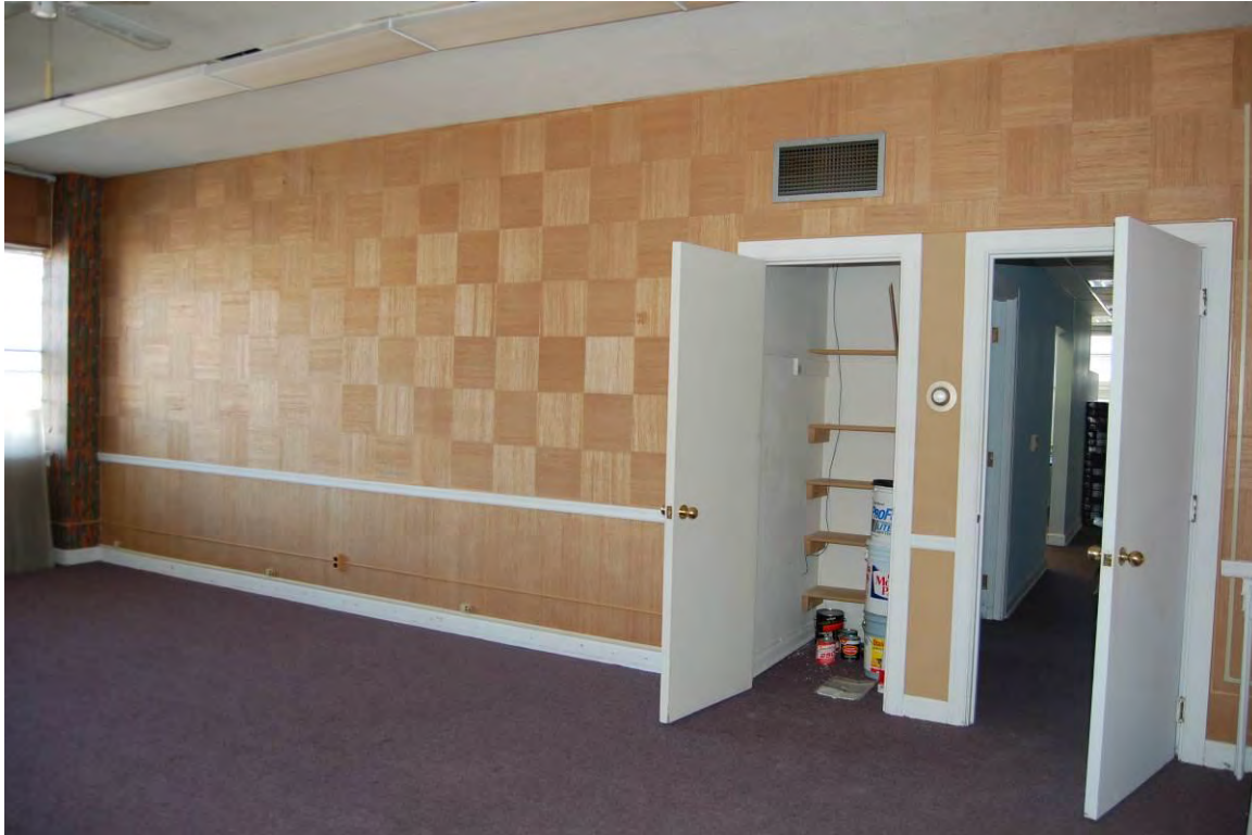
Figure 3. This area, currently used for storage (Photo 2012) illustrates an original wall finish and carpeted terrazzo floor.
