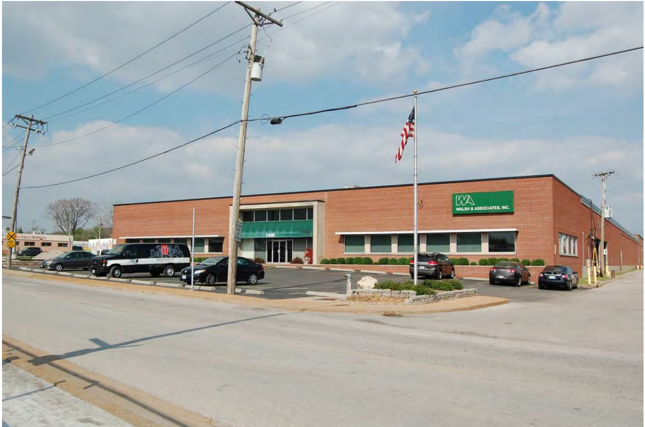
Figure 14. 1400 Macklind Avenue, view is northeast.
