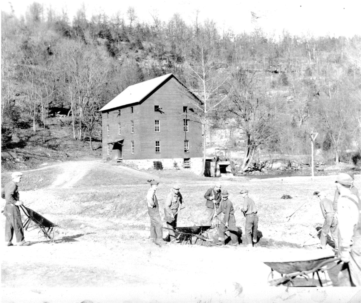
Figure 26. Men working on the flood control channel, which involved changing the course of Alley Hollow Creek away from the south side of the mill. February 1934. (Ozark National Scenic Riverways catalog number OZAR 24060.)
