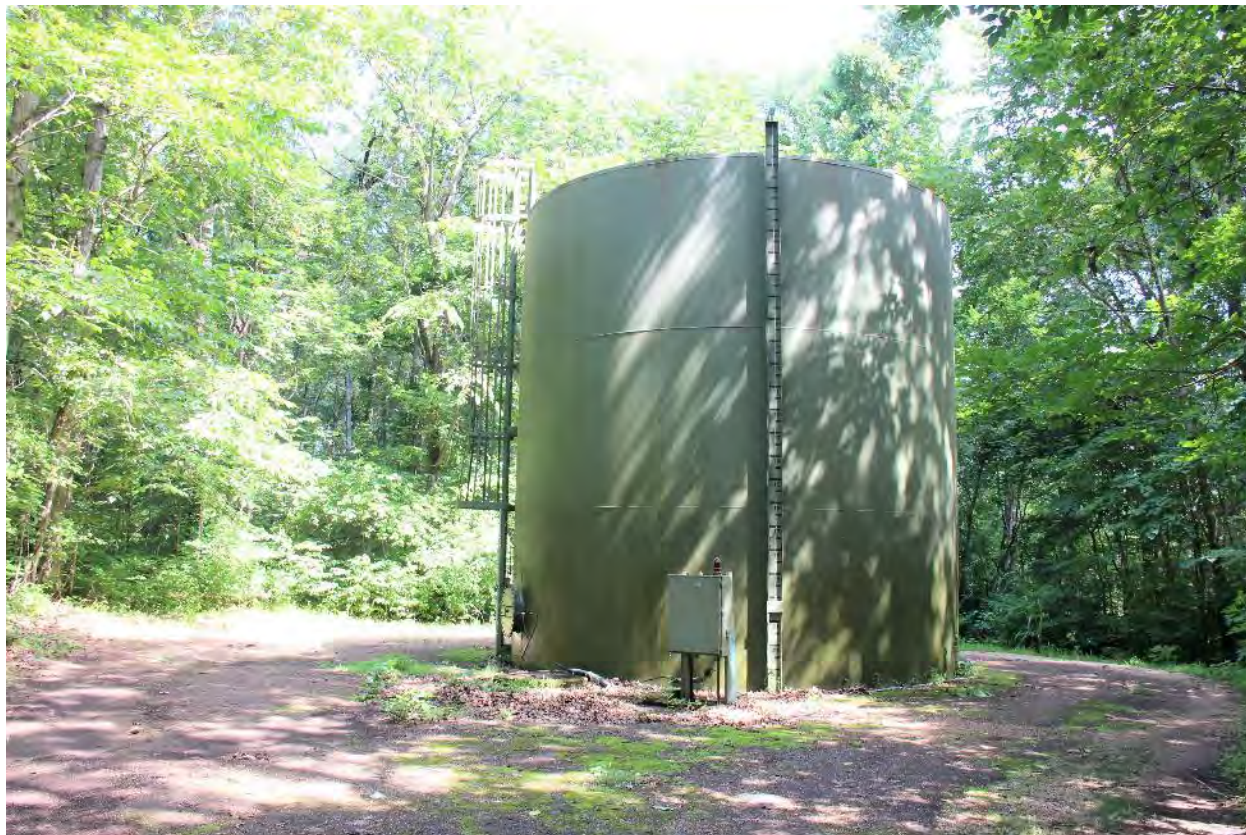
Photo 20. Water tower. Camera facing northwest. (Deb Sheals, 2019.)
