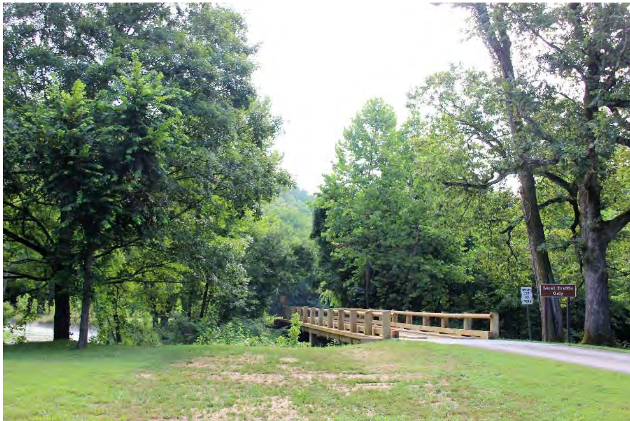
Photo 11. Alley Spring Branch Vehicular Bridge. Camera facing east. (Deb Sheals, 2019.)
