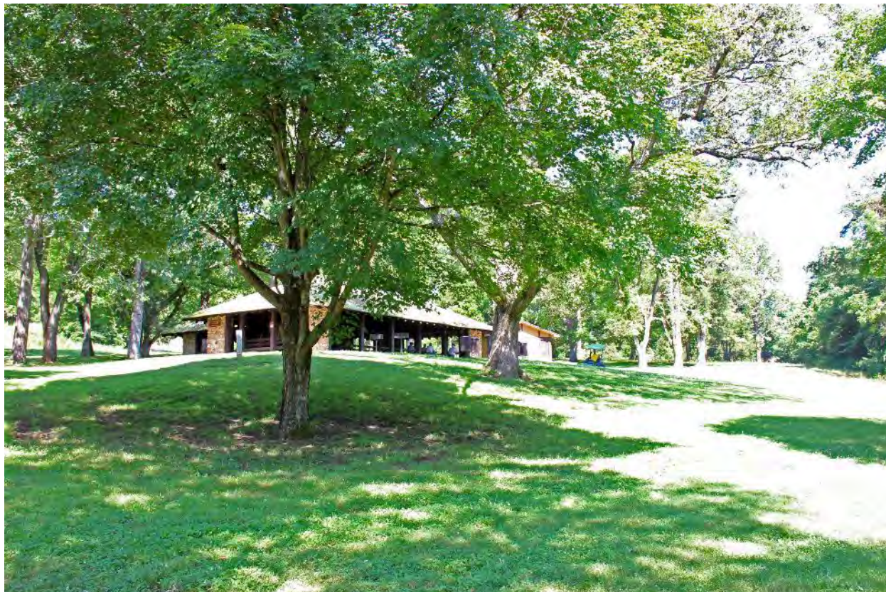
Photo 7. Alley Spring Picnic Shelter and restroom. Camera facing north. (Deb Sheals, 2019.)
