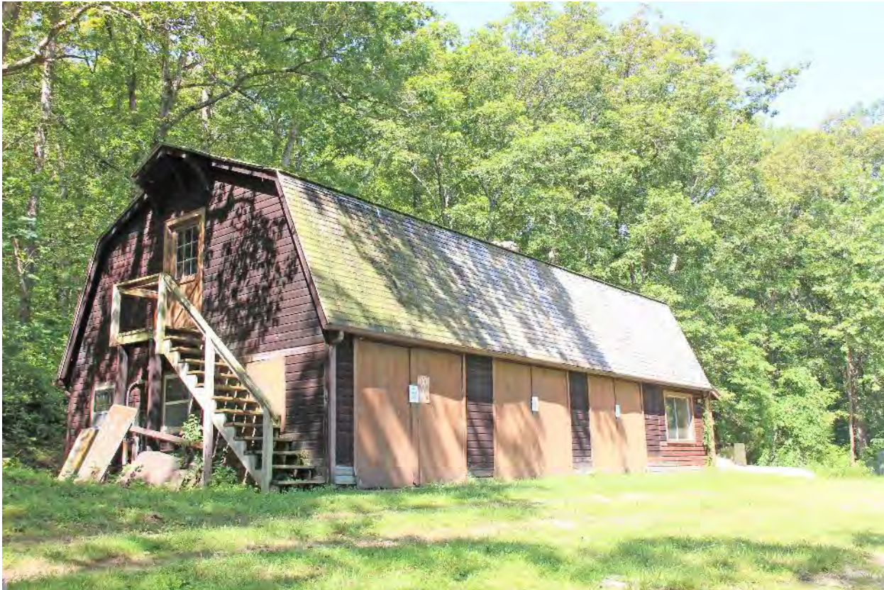
Photo 16. Alley Spring District Maintenance Shop. Camera facing west. (Deb Sheals, 2019.)
