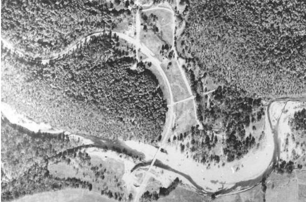
Figure 29. Aerial photo of Alley Hollow, 1955. (Curtesy of Dan Jackson, National Park Service.)
