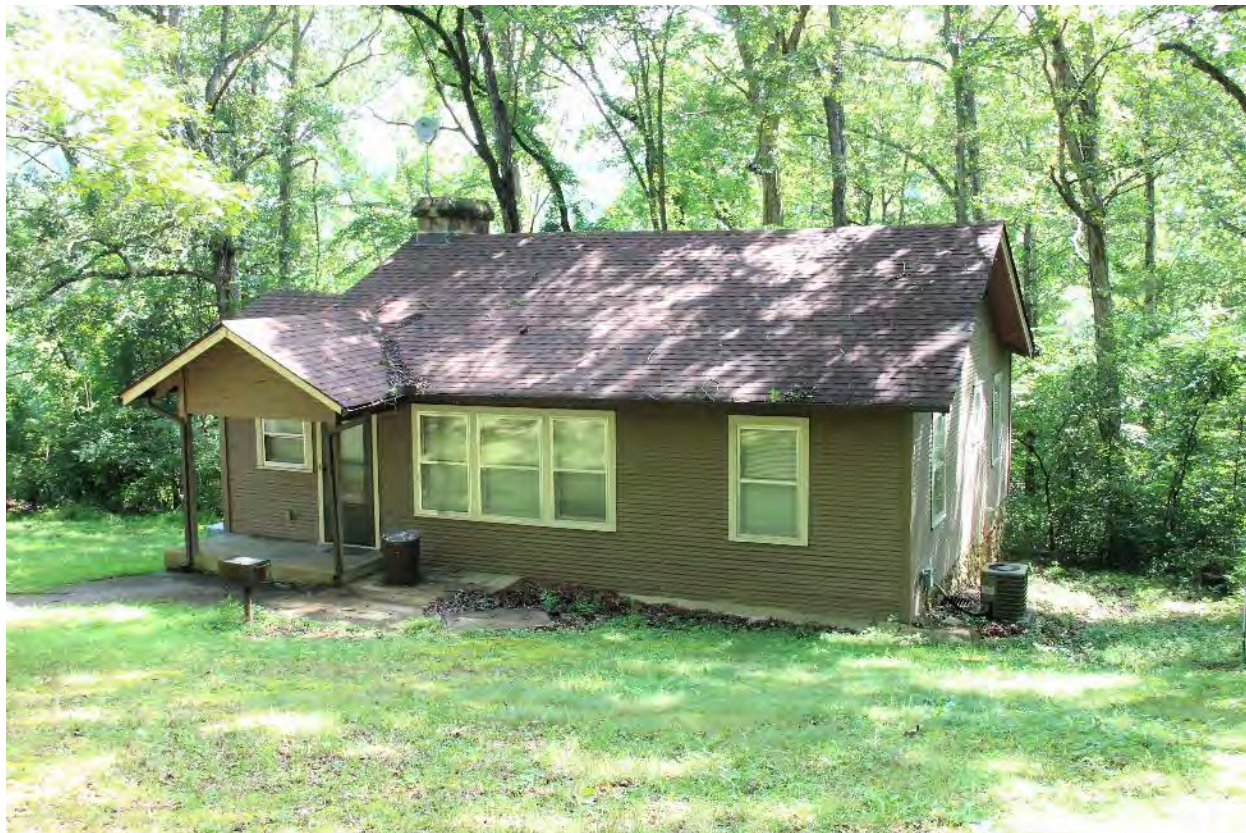
Photo 17. Park Keeper's House. Camera facing northeast. (Deb Sheals, 2019.)
