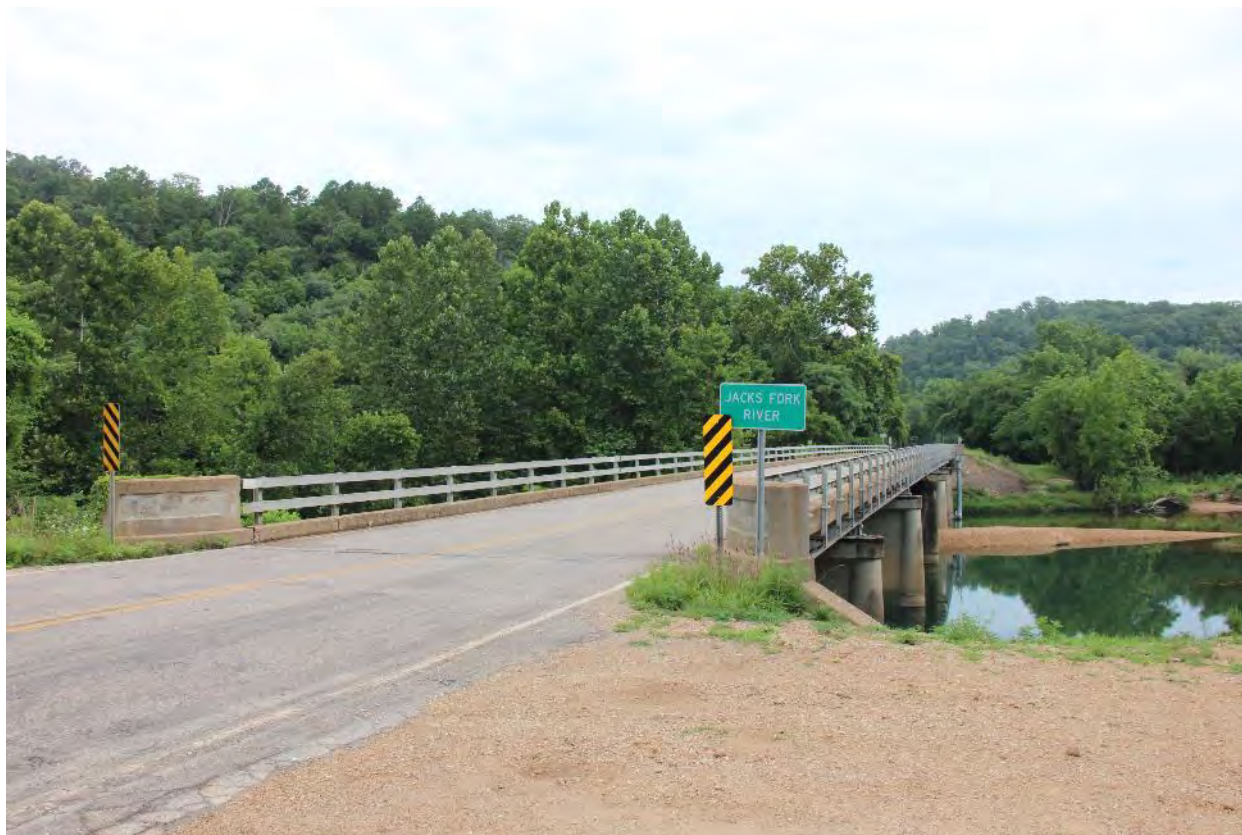
Photo 22. Jacks Fork Vehicular Bridge. Camera facing north. (Deb Sheals, 2019.)
