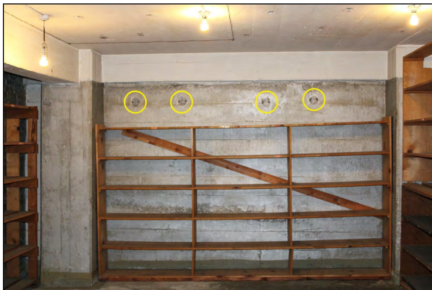
Figure 22: (Top) Entry doors to narrow vault at the basement level, 2022. (Bottom) Narrow vault interior, basement level. The yellow circles highlight the location of mounts for valet rods, 2022. Source: Kelsey Lutz, photographer.
