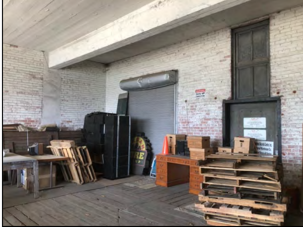
Figure 25: Dock area at the south elevation with original rolling fire shutters and hinged steel-clad fire door, 2022.
