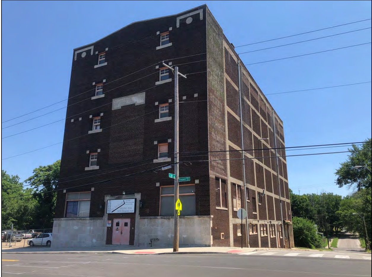
Figure 21: The former Perky Brothers Transfer and Storage Company, constructed in 1913 and located at 2431 Prospect Avenue, Kansas City, Missouri, 2022.
