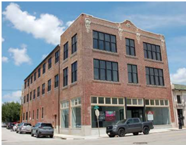
Left: The Tate Motor Car Company Building before rehabilitation (2022); Right: After rehabilitation (2024). The original windows had been infilled with glass block, and the storefront had been concealed under painted metal panels. The rehabilitation returned historically compatible windows and storefronts to the building.
