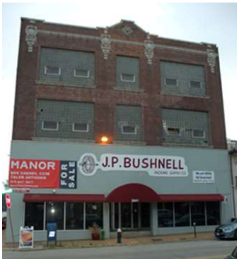
Left: The Tate Motor Car Company Building before rehabilitation (2022); Right: After rehabilitation (2024). The original windows had been infilled with glass block, and the storefront had been concealed under painted metal panels. The rehabilitation returned historically compatible windows and storefronts to the building.
