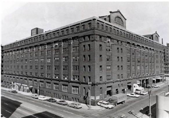
Left: The Butler Brothers warehouse in the 1950s.
