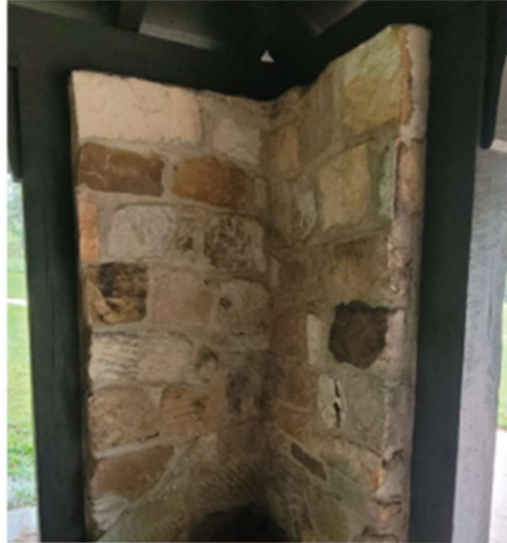
Exterior (left) and interior (right) of an Ozark rock masonry support wall of the Alley Pavilion at the NPS Alley Spring campground. The photo on the right shows typical "giraffe" construction with flat sandstone slabs.
