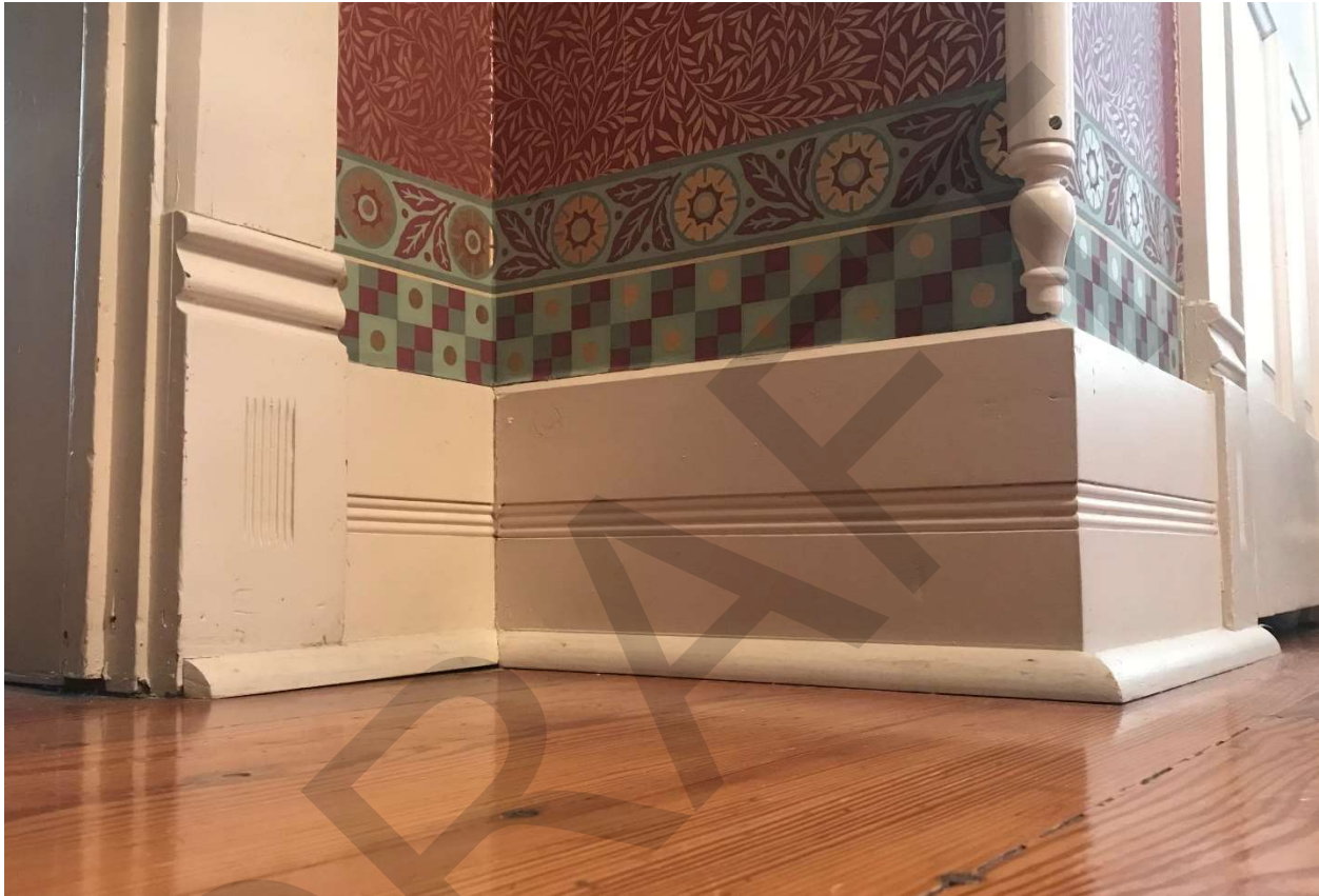
Figure 12: Typical Second Floor Trim, Baseboard and Door.
