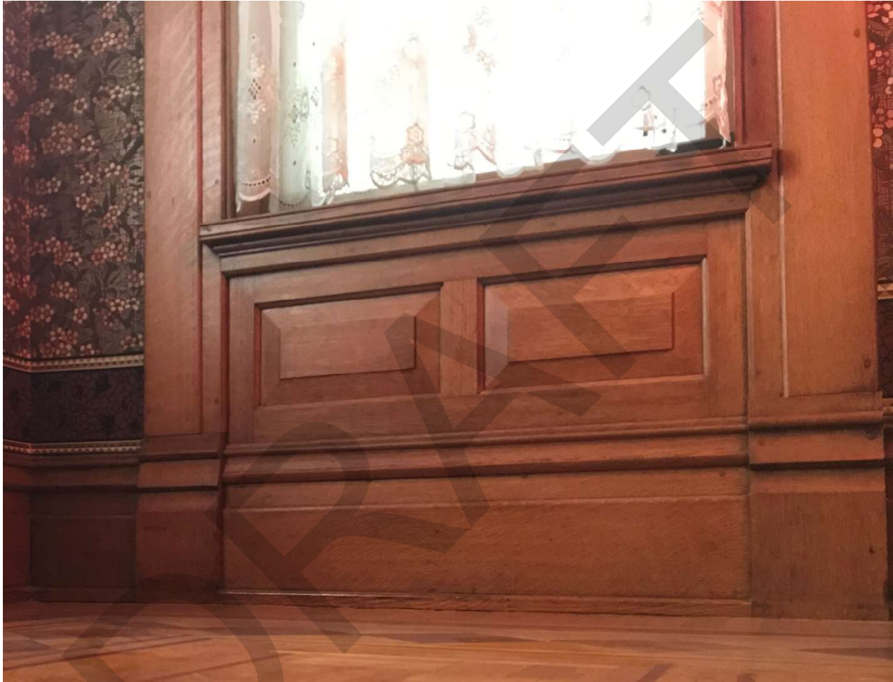
Figure 10: Typical First Floor Trim, Windows and Baseboard.
