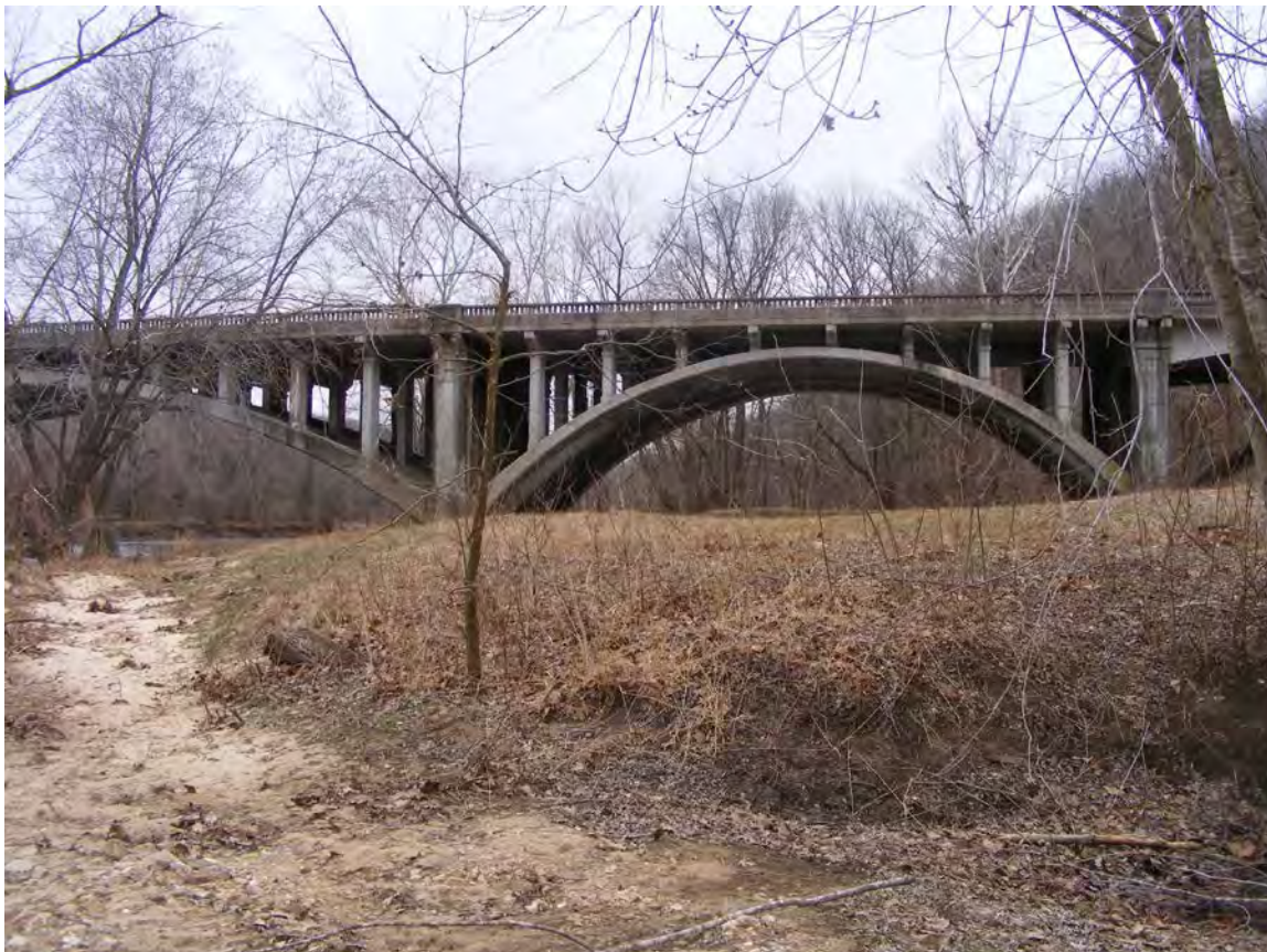
Figure 5. Piney Beach Bridge, view is northeast. Photo: Ruth Keenoy, 2014.
