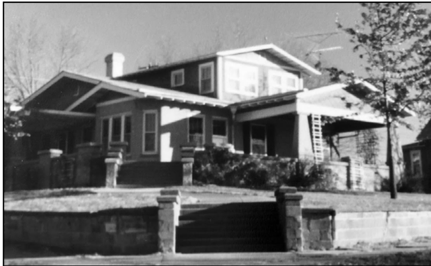
FIGURE I: The Fields Home, late 20th century. Notice the exposed rafters under the eaves. Photo courtesy of Jill Chadwick.
