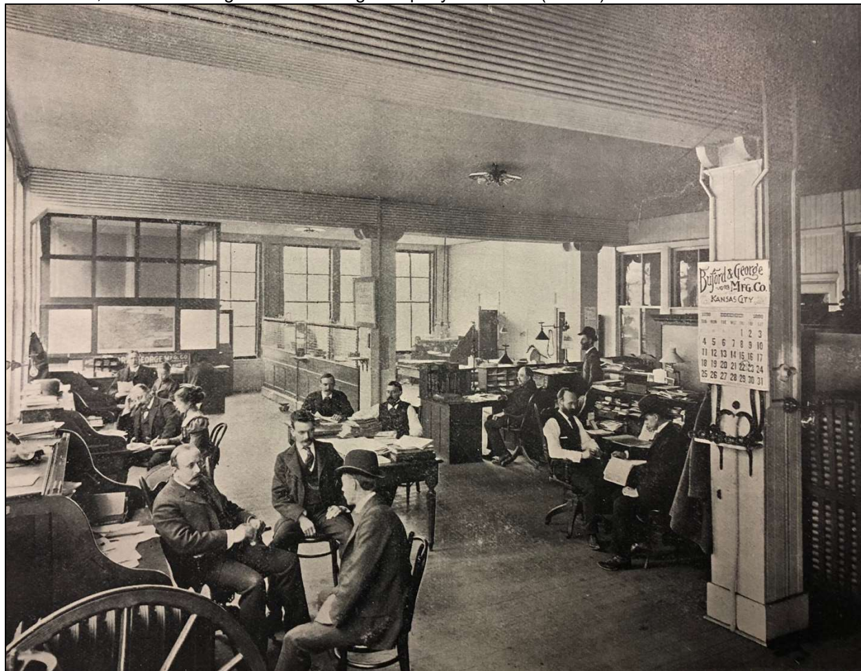
Figure 13: 1311-1315 W. 13 th Street, Interior. Offices, 1st floor, 1898 (view looking southeast). The entry partition as seen in the background of this image was not illustrated on the original drawings.
