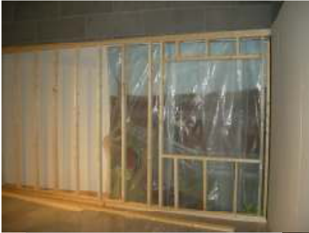
Start of the framing for the new Civil War Exhibit
