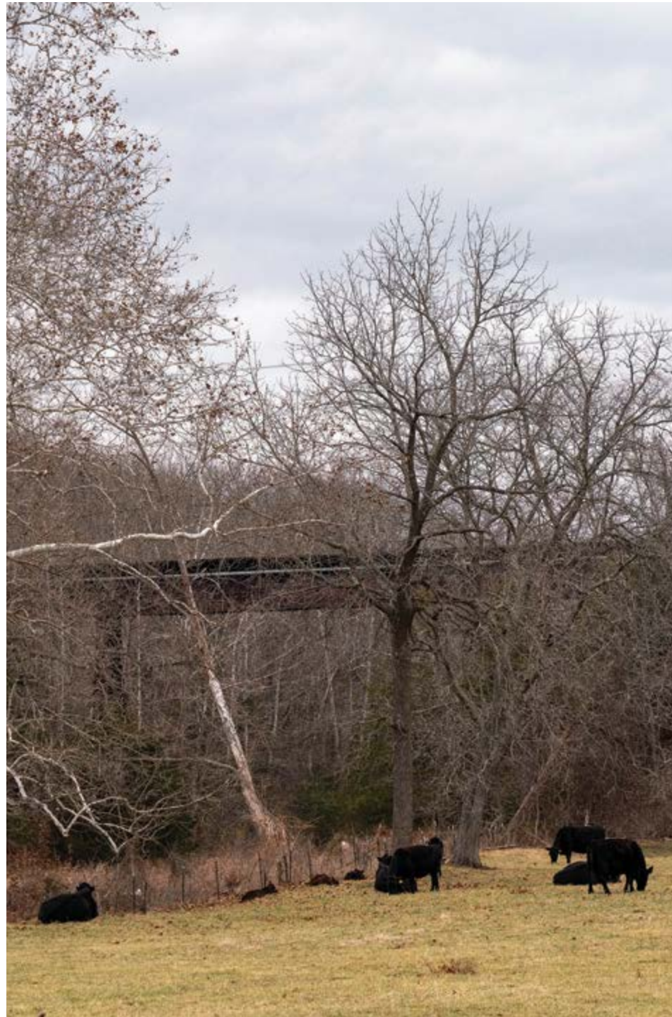
Soap Creek Bridge
