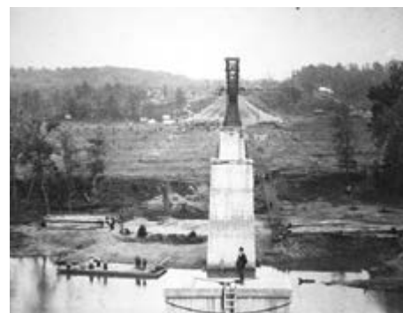
Rock Island Railroad bridge construction
