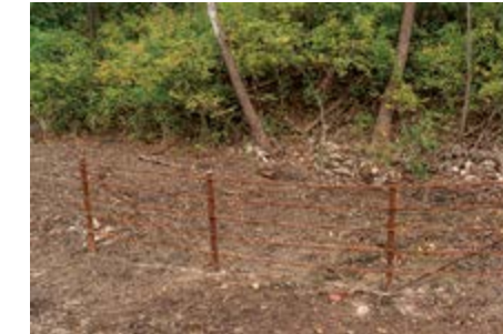
Completed fencing project in Miller county
