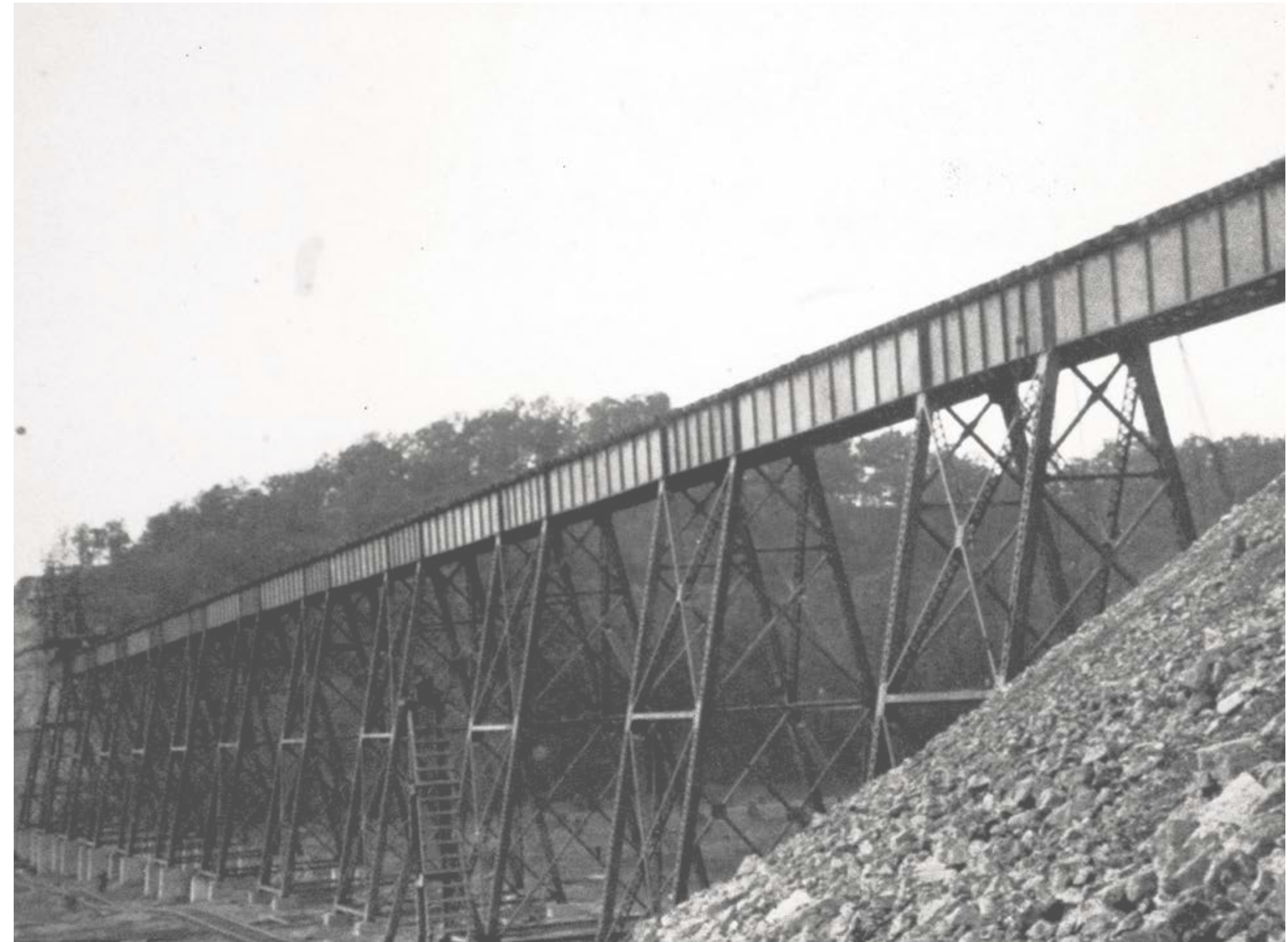
East side approach to Gasconade River bridge. Circa 1902.
